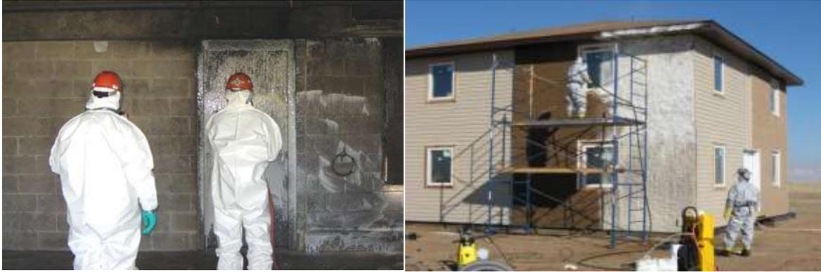
Building decontamination using Rad-Release foam to quickly cover large surface areas
